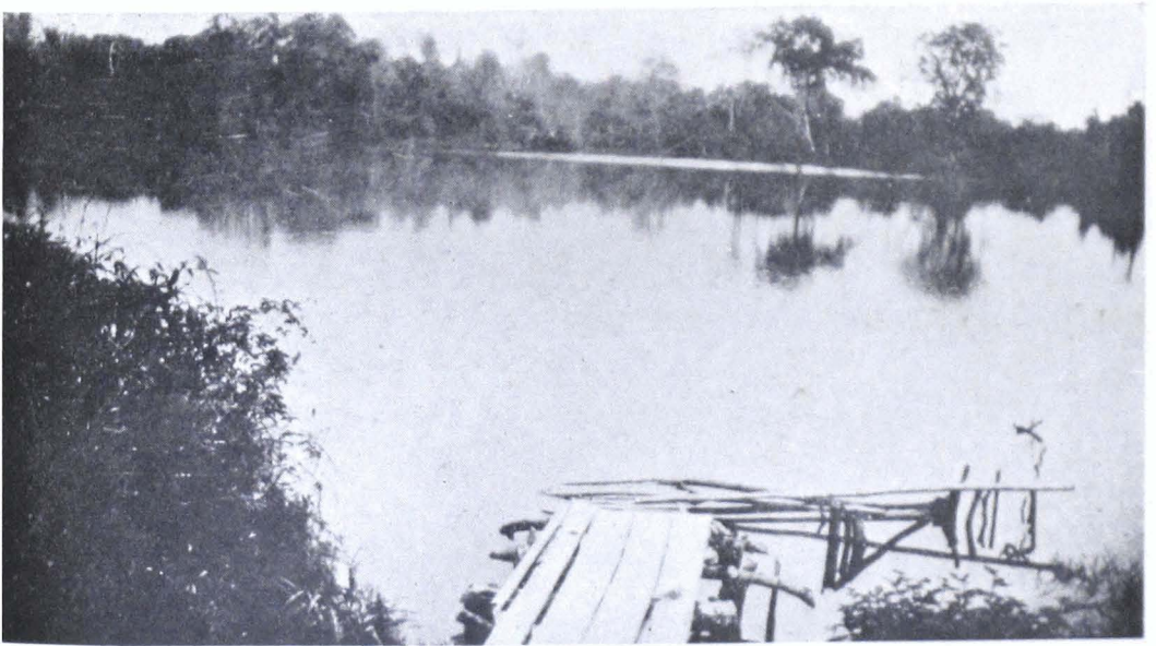
ONE OF THE LARGE EXCAVATED TANKS AT DIMAPUR, IN THE NAMBHOR FOREST.
